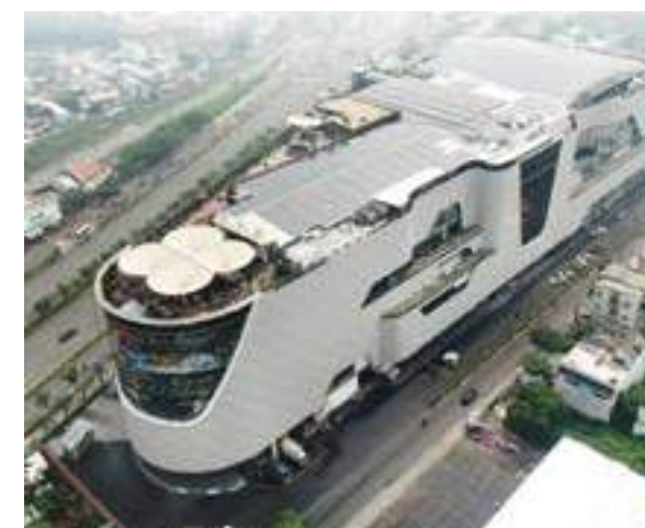
GIGA MALL 517,48 kWp
